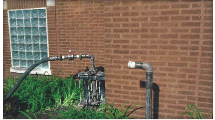
Pipes driven adjacent to exterior walls.
