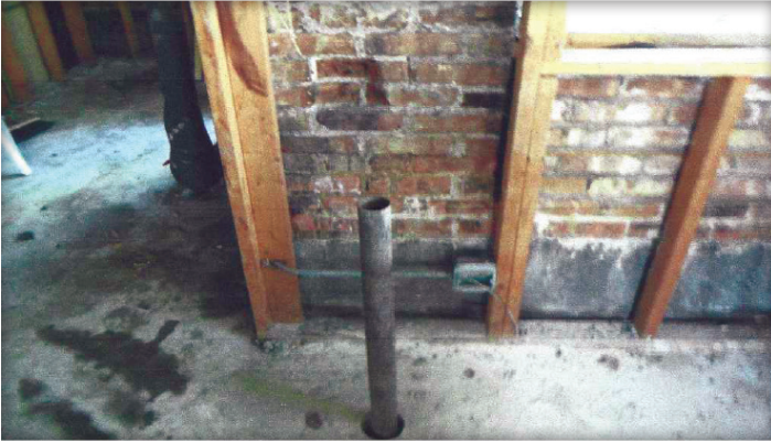
Coring 3-inch diameter holes through the basement floor.
